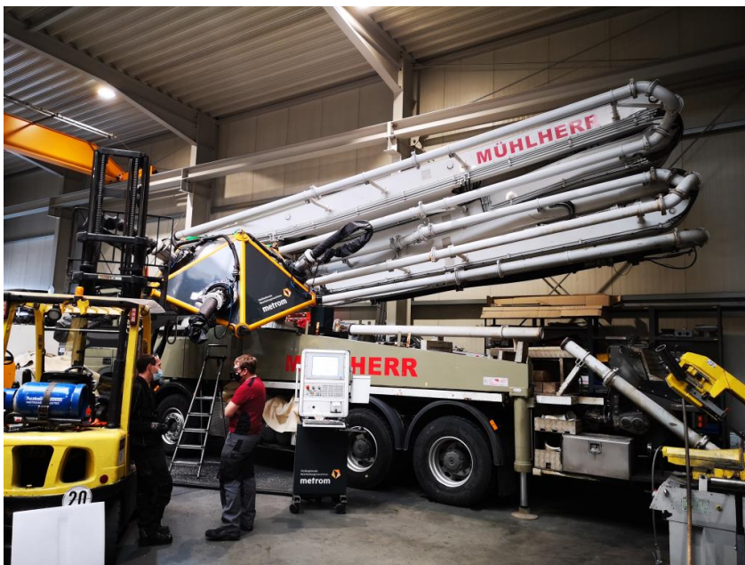
Figure 4 Milling out jammed boom bolts on a mobile concrete pump
