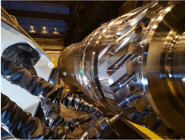
Figure 3 Modification of a gas turbine at the customer's plant on site
